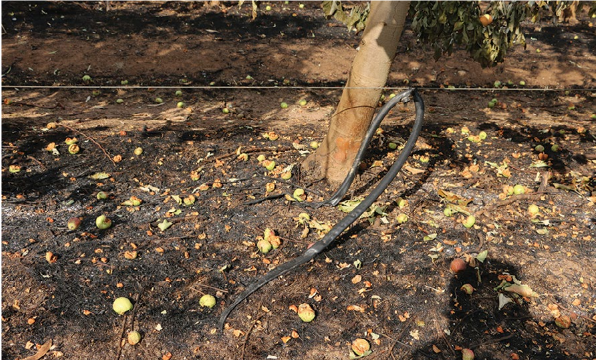
Figure 22. Low-density polyethene irrigation tubes that supply irrigation to trees via dripper or sprayer were exposed to fire damage.
